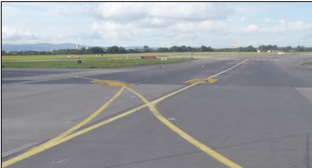
Photo No. 1: New Taxiway Directional Pavement Markings Installed at Link 2
